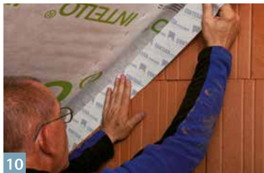
CONTEGA SOLIDO SL Forms adhesive bonds with mineral substrates, can be plastered over; ensures reliable, airtight joints with substrates that are to be plastered over for all building trades
