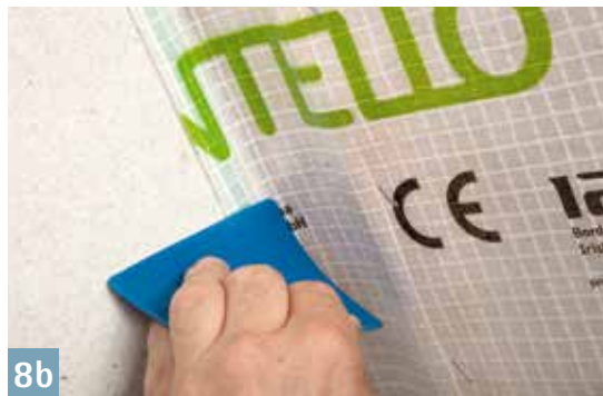
ORCON MULTIBOND Creates reliable joints with rough or mineral adjacent building components; joints can be subjected to loading immediately
