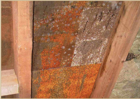
Fig. 44. Mould in the building envelope
