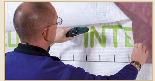
Fig. 86. Taping overlaps
