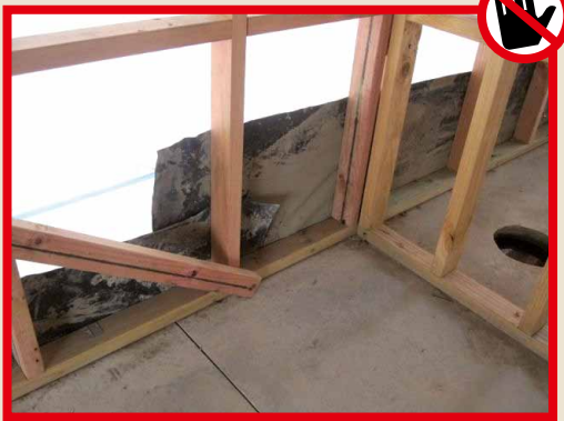
Fig. 79. Bitumen membrane outdoors
