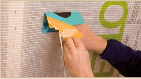
Fig. 90. ROFLEX pipe grommet fixed with TESCON VANA
