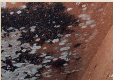
Fig. 3. Mould in the building structure
